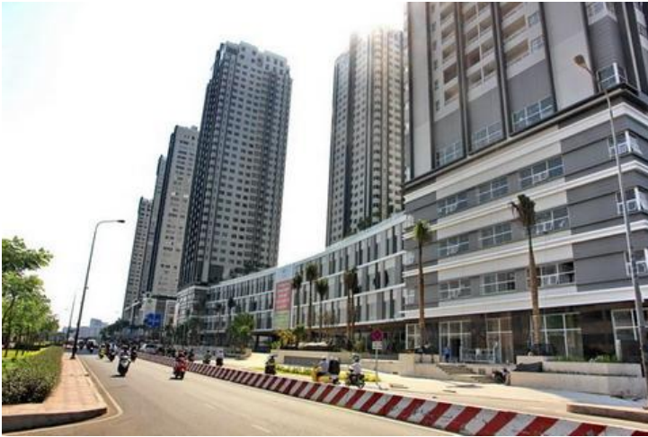
A high-rise boom in ever-growing HCM City is posing new management challenges for authorities, a construction official reported on Monday
